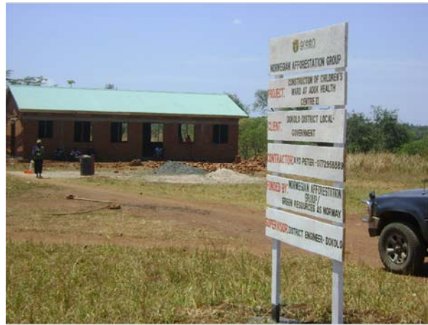
Figure CM.1.1.2 Construction of the children's ward at the health centre II
